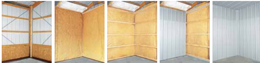
View of corner section before insulation
