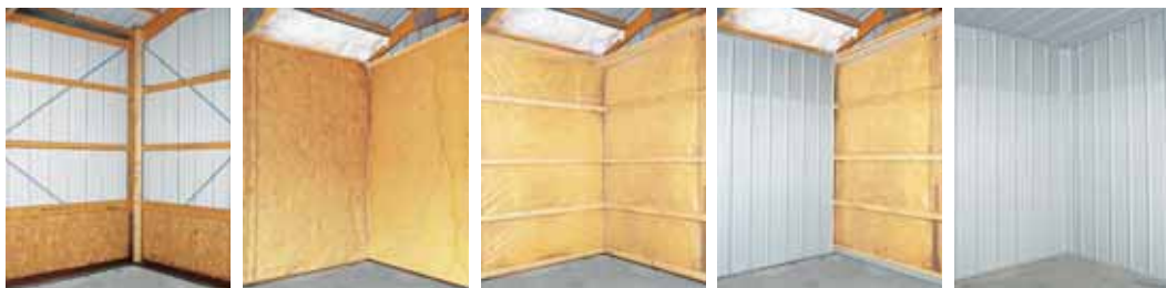
View of corner section before insulation
