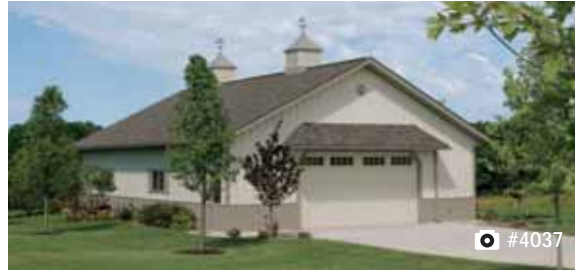
Garage & Residential Storage
