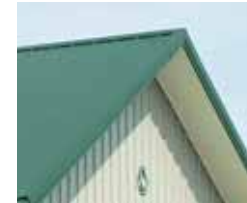
Non-Vented Soffit
