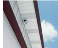
Vented Soffit
